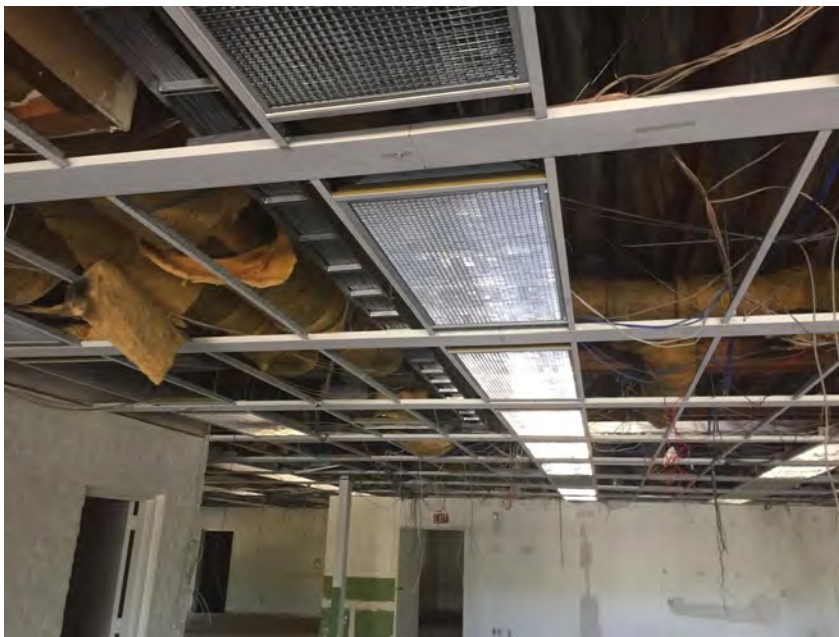
Figure 2-6 Typical Office Ceiling
