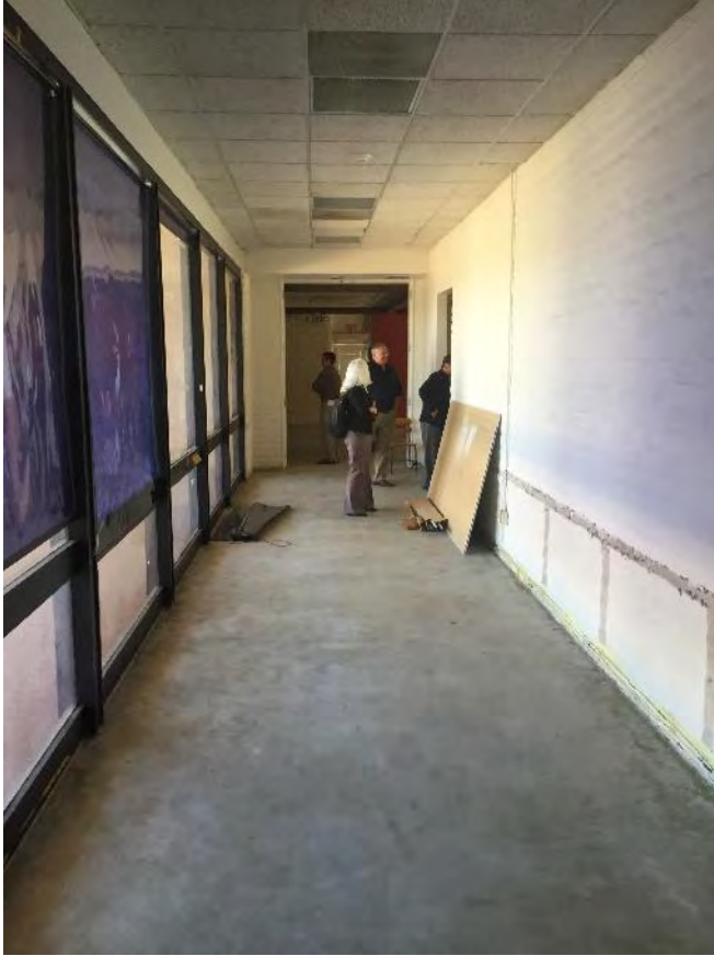
Figure 2-3 Hallway from the Front Entrance to Board Room (looking north)
