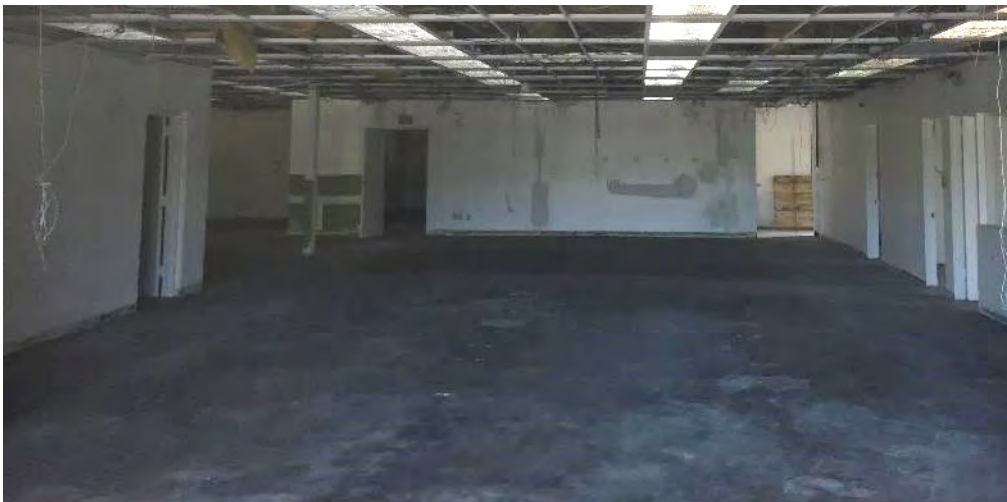
Figure 2-5 Existing Building Open Space (looking east from near the front entrance)
