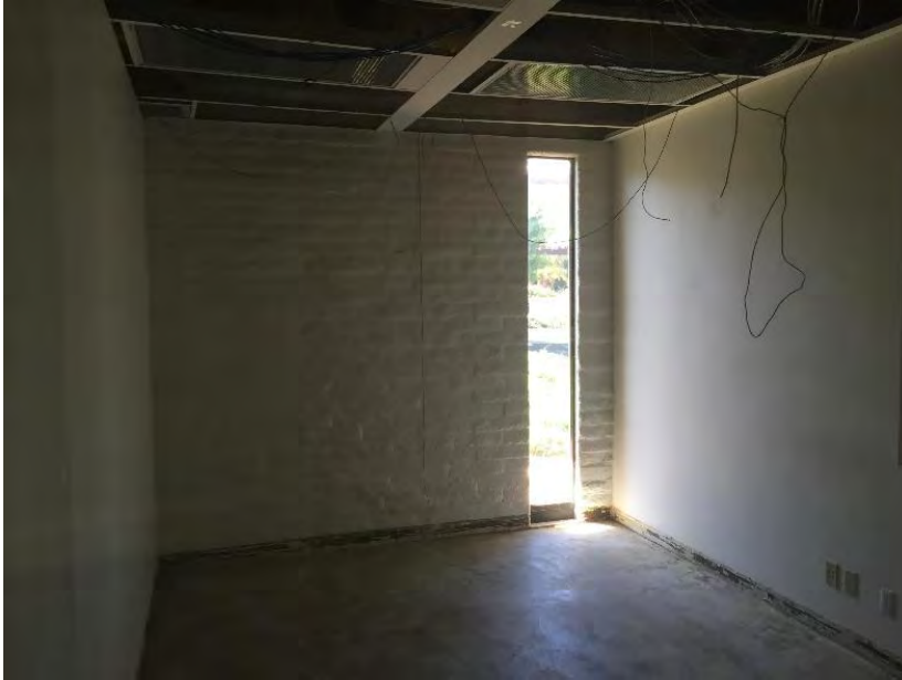
Figure 2-8 Existing Building Office
