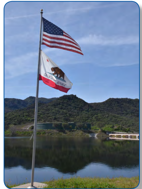
The 5 million gallon tank built at Las Virgenes Reservoir was a major part of the potable water backbone improvement program.
