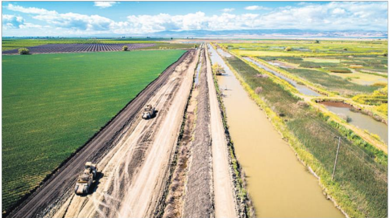
EARTH MOVERS carry dirt to shore up levees at the Kings River and Fresno Slough. If the levees fail, farmland would be inundated.
