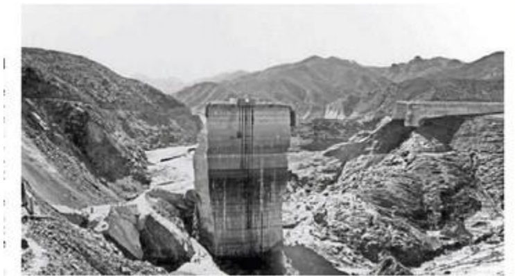
This photo was taken in 1928, days after the St. Francis Dam collapsed east of Santa Clarita. STAR FILE PHOTO
