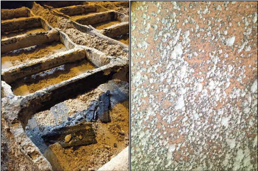
Figure 8 Interior Corrosion in Bulk Amendment Bin
