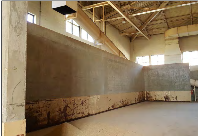
Figure 4 Existing Conveyor System and Reserve Amendment Storage Area
