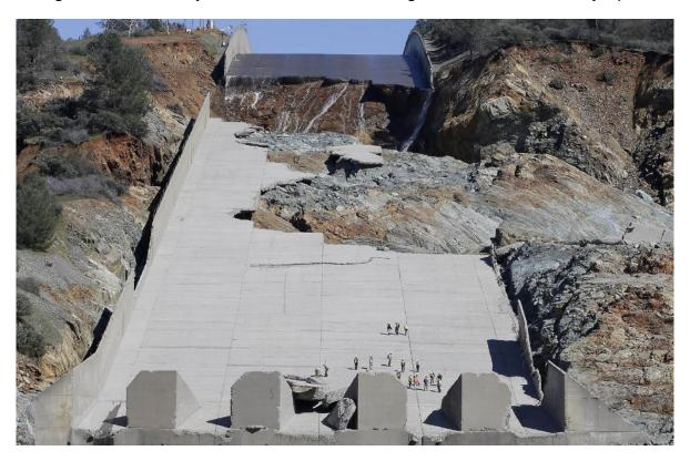
OFFICIALS SURVEY massive damage to the Oroville Dam's main spillway in February. The state's plans call for replacing portions of the upper chute by Nov. 1 in order to prepare the reservoir for the next rainy season. (Photographs by Rich Pedroncelli Associated Press) CREWS dredge the riverbed near the spillway, where repairs are likely to exceed a \$200-million estimate. ()
