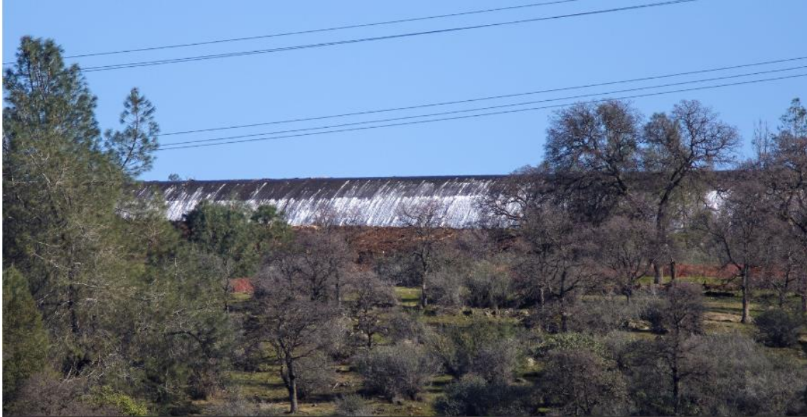
BLOATED with storm runoff, the Lake Oroville reservoir had gone from 80% full to overflowing in less than a week when managers were forced to reduce releases on the dam's heavily damaged concrete spillway. (Brian van der Brug Los Angeles Times)
