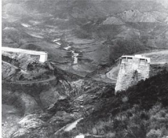
This aerial view shows the broken water barrier of San Francisquito Canyon after the St. Francis Dam burst in 1928. PICASA, AP
