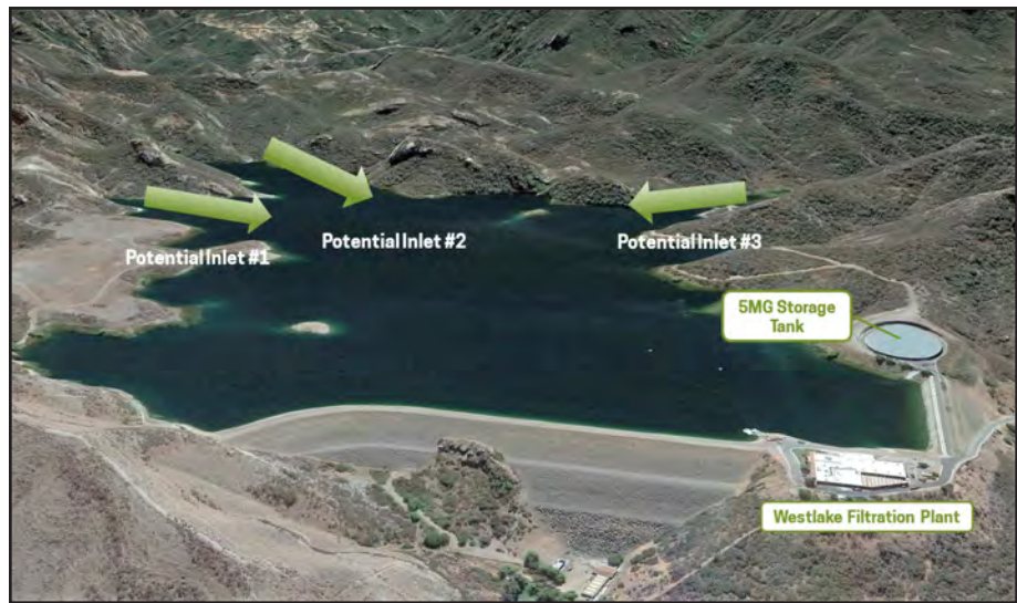
RMC has identified three preliminary inlet locations at LVR based on the reservoir configuration, the location of existing recycled water pipelines, and distance to the existing outlet structure near the Westlake Filtration Plant.
