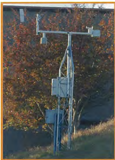
Figure 4. Meteorology station at Las Virgenes Reservoir
