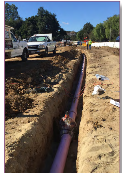
Agoura Road 8" Recycled Water Main Line Extension
