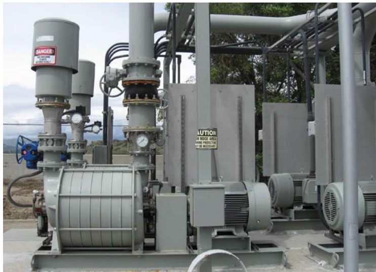
Figure 4.1 Typical Multi-Stage Blower Installation
