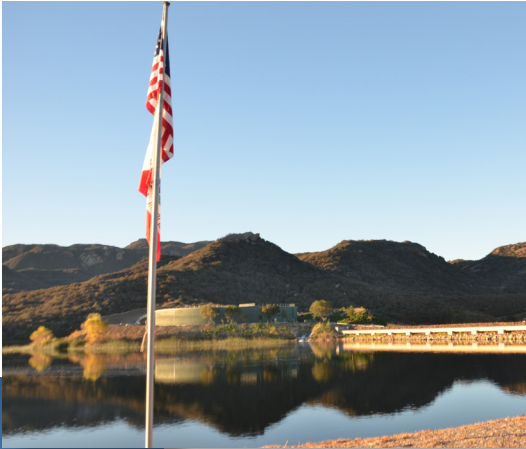
5-million gallon storage tank at Las Virgenes Reservoir, completed in 2015.
