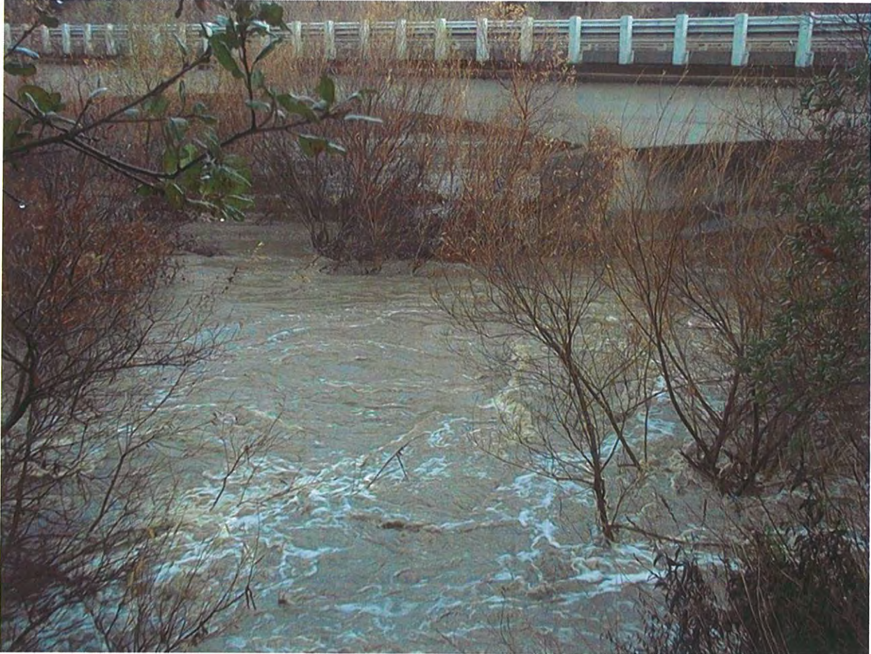
January 10, 2005 Malibu Canyon Bridge top of the pier is at elevation of 465 feet. Peak Flow 12,700 cfs.
