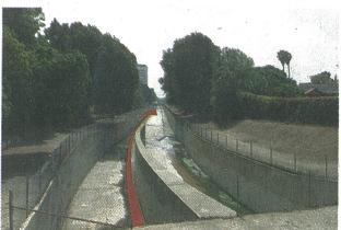
The cigarette butt travels further south, washing back underground and into pipes heading toward Ballona Creek. The U.S. Army Corps of Engineers lined the creek with concrete as part of the creation of the storm drain system in the 1930s and 1940s. Screens and nets have since been installed to catch some of the trash before it gets to the ocean.
