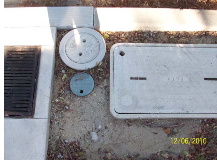
Utilities on Park Capri
