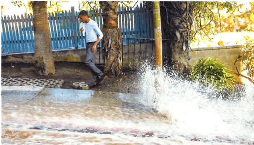
In September, water gushed along North Olive Drive in West Hollywood after a pipe broke. (Jay L. Clendenin / Los Angeles Times)
