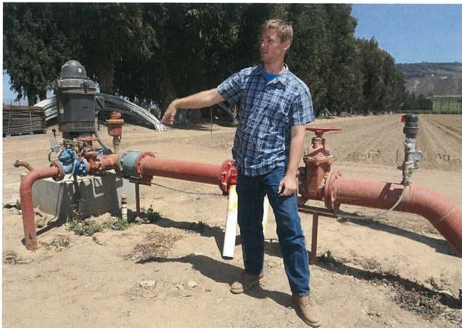
ROB VARELA/THE STAR Jason Vis explains how a groundwater pump automatically turns on based on water levels in storage tanks at Lloyd-Butler Farms near Saticoy.
