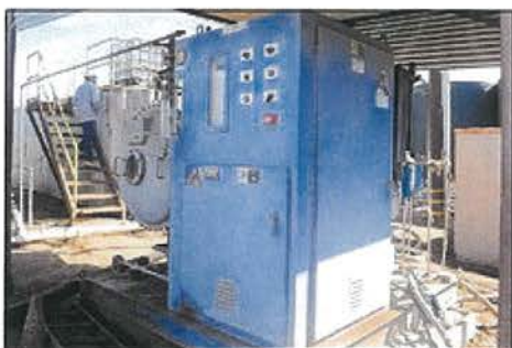
Carl Edwards, vice president sales and marketing, looks at one of the holding tanks at Southern California Waste Water in Santa Paula.
