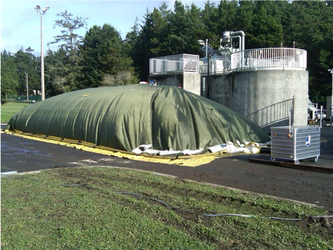
Figure 4-3: Example Static Pile Installation for Potential Piloting at Rancho
