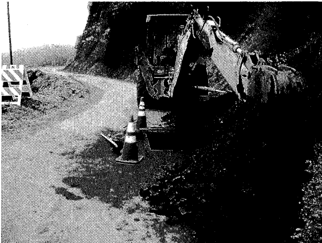
Barrymore Leak Site - Photographs
