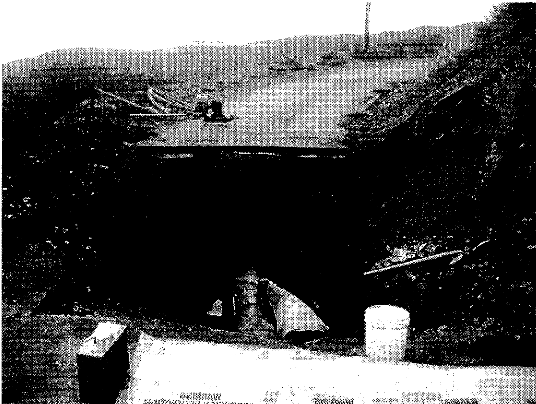
Barrymore Leak Site - Photographs
