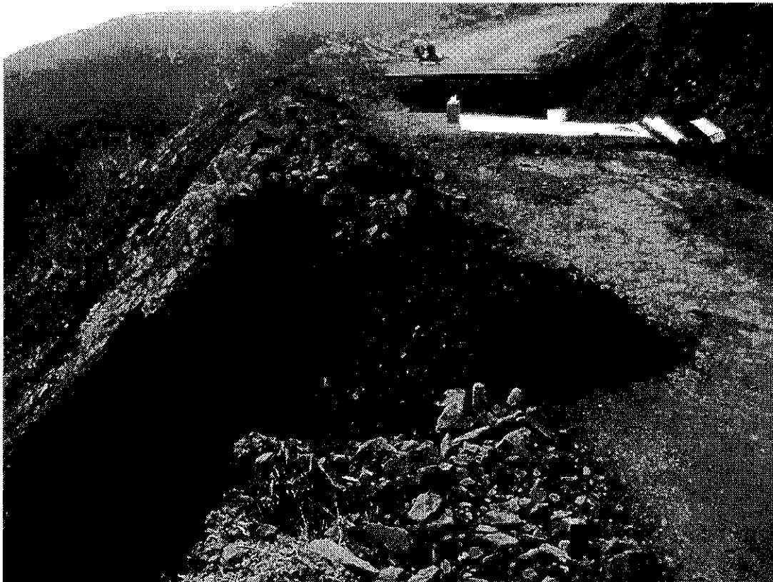
Barrymore Leak Site - Photographs
