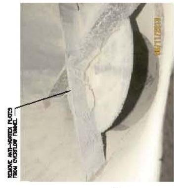
ANTI-VORTEX PLATES SCALE: ITS
