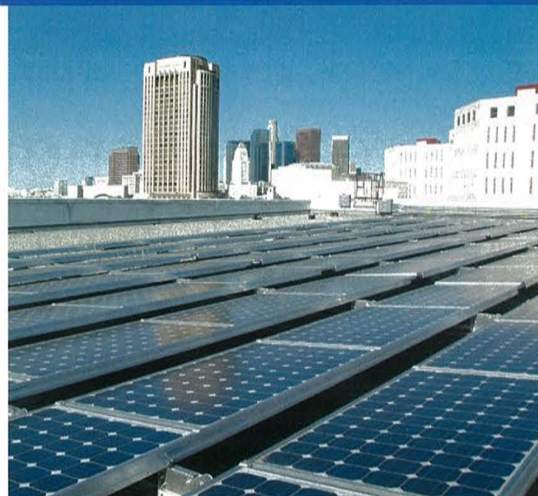
Solar panel collectors at Metro facilities in downtown Los Angeles.
