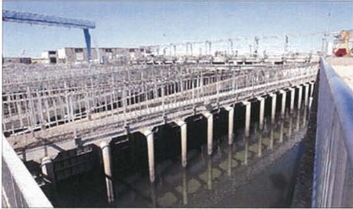
Water flows through fish diversion louvers at the John E . Skinner Delta Fish Protective Facility from the Clifton Court Forebay on its way to the Harvey O. Banks Pumping Plant.
