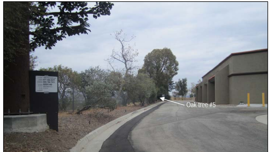
Photo 4. View looking east along northern boundary of the Plant. The proposed limit of work adjacent to the protected trees is the existing access road's curb.
