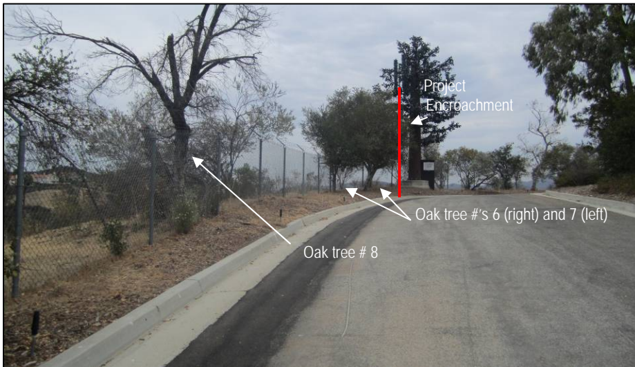
Photo 3. View looking north along western edge of the Westlake Filtration Plant. Project encroachment is delineated by red line at edge of Oak tree #6's canopy.
