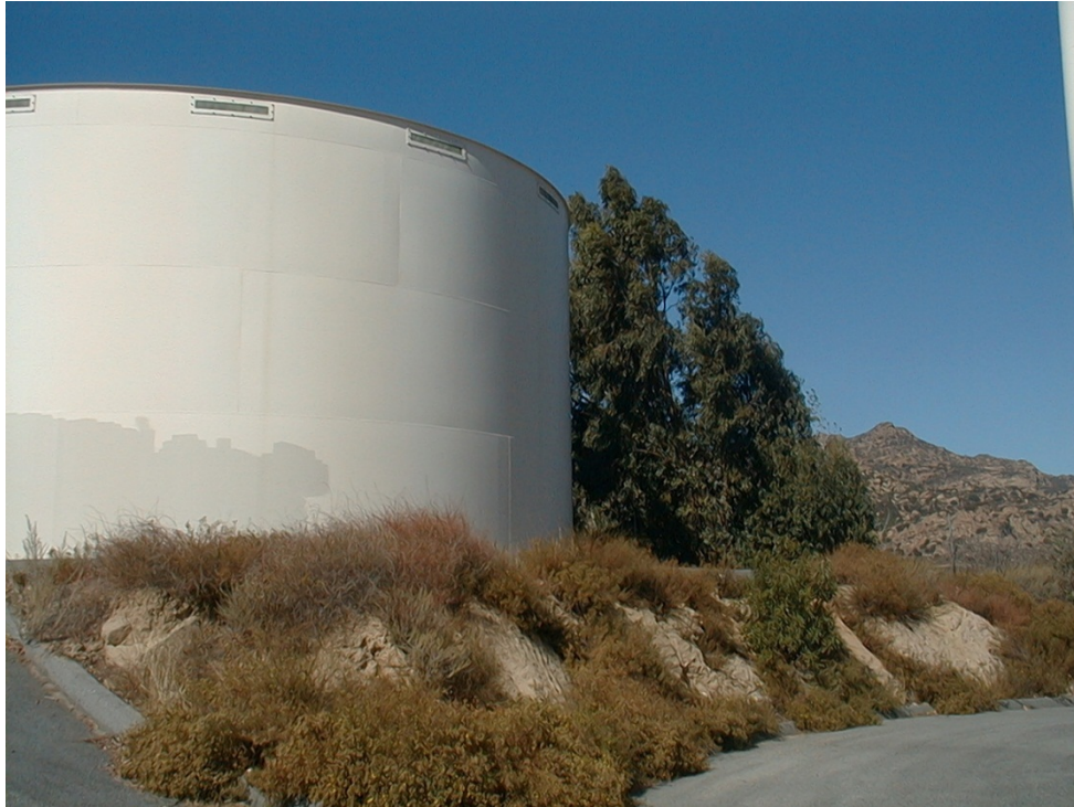
Figure 28—Twin Lakes Tank Site
