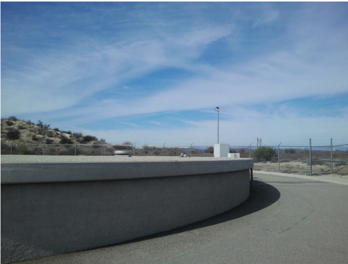
Figure 12—Existing control panel with antenna
