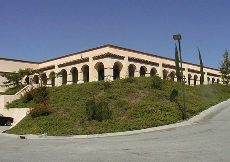
Figure 2—Filtration building corner where antenna will be placed
