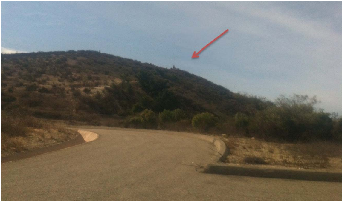
Figure 35—View of 20 foot pole from the driveway leading up to Lower Oaks Tank
