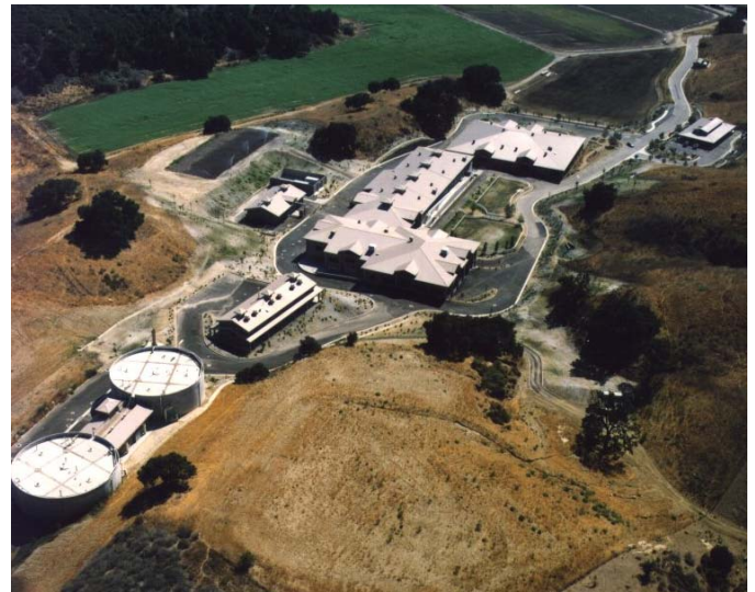
Figure 11—Aerial view of Rancho Composting Facility facing south
