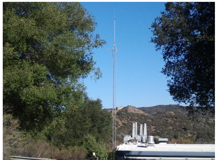
Figure 18—Tapia Antenna Tower from front of control building (close up)
