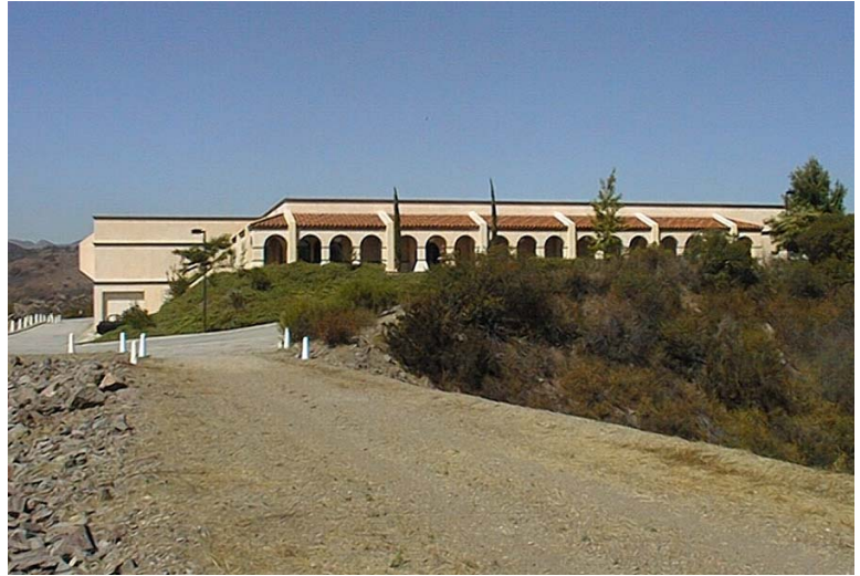
Figure 3—Westlake Filtration Plant
