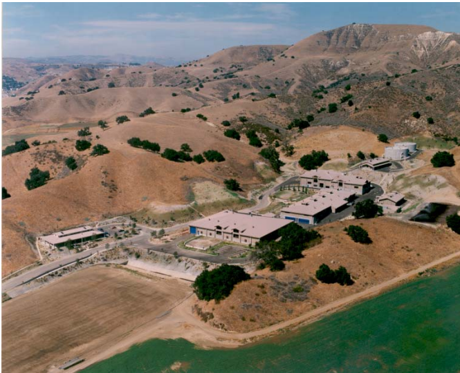
Figure 10—Aerial view of Rancho Composting Facility facing northeast
