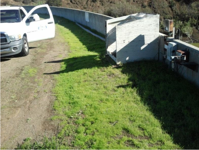
Figure 19—Tapia Repeater Tower location by Reservoir 1 air compressor
