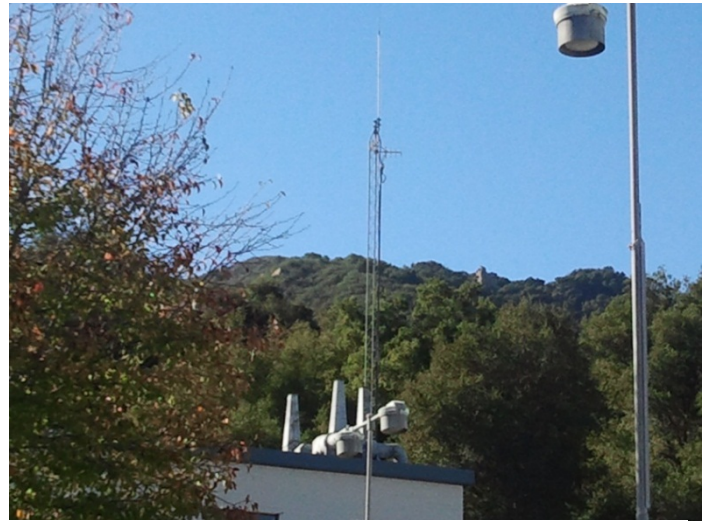
Figure 16—Tapia Antenna Tower from back of control building (close up)
