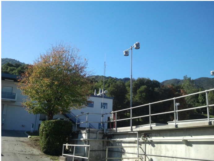
Figure 15—Tapia Antenna Tower from back of control building (wide angle)
