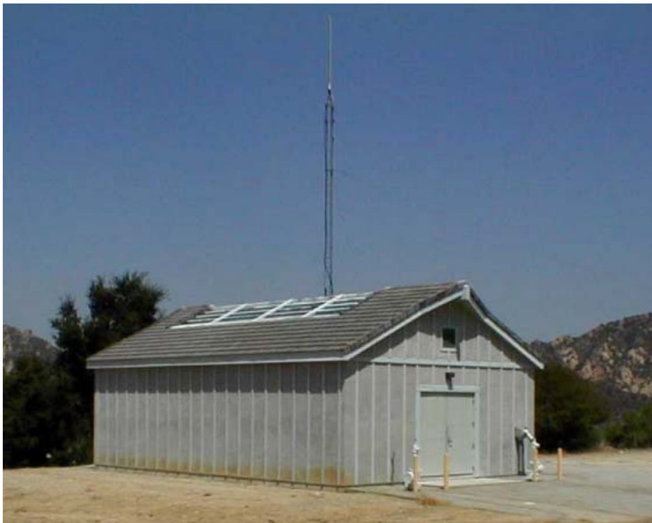
Figure 25—Stunt Road Pump Station
