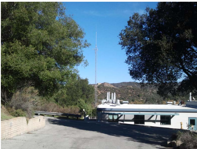
Figure 17—Tapia Antenna Tower from front of control building (wide angle)
