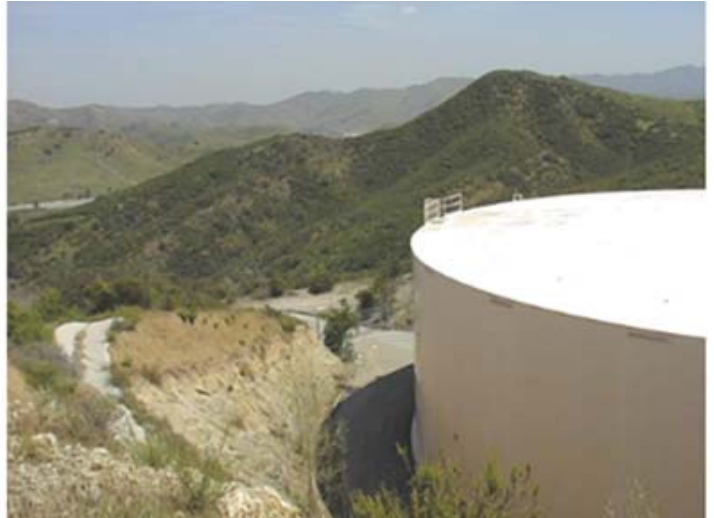
Figure 30—Indian Hills Tank Surrounding Area
