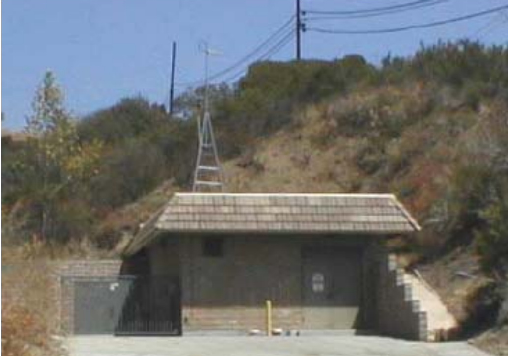
Figure 27—Cold Canyon Pump Station
