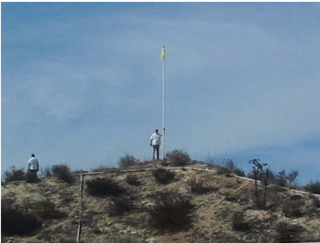
Figure 34— Twenty foot pole at proposed antenna location, facing northwest at Lower Oaks Tank
