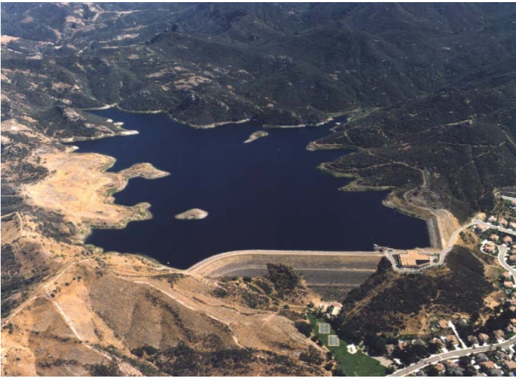
Figure 4—Aerial view of Westlake Filtration Plant
