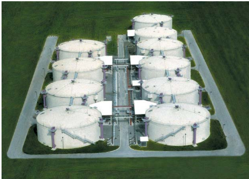
FIGURE 2-9 FIXED CONCRETE DOME COVER
