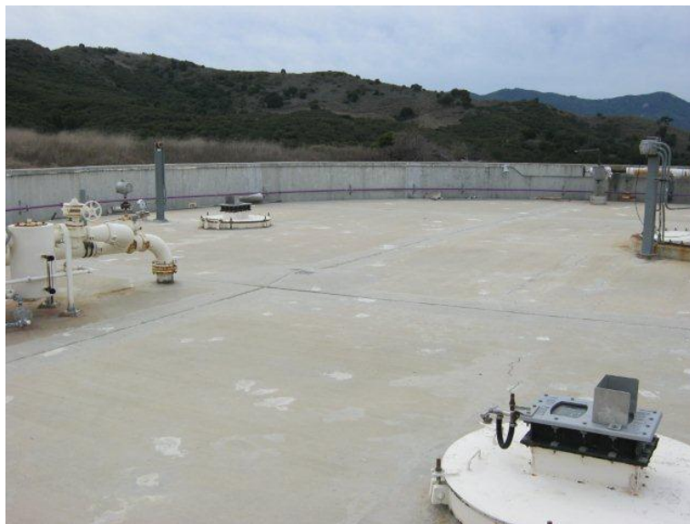
FIGURE 2-8 FIXED CONCRETE FLAT COVER
