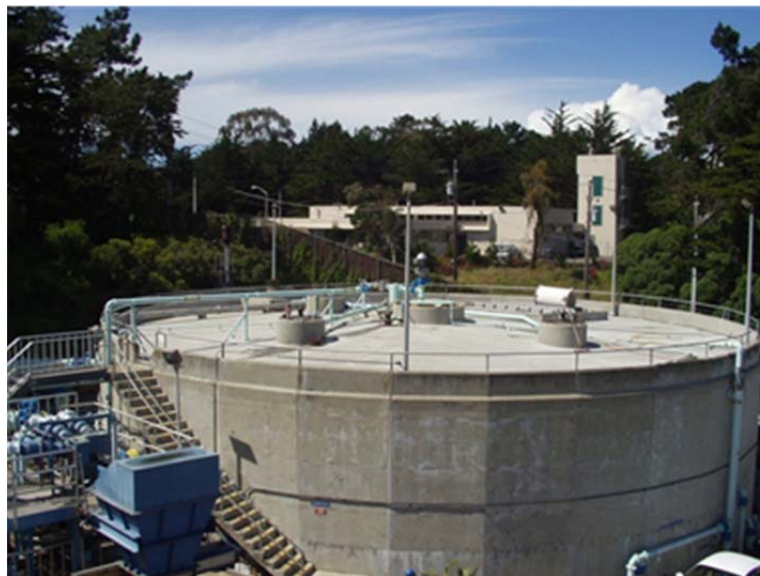
FIGURE 2-10 FINISHED FIXED FLAT CONCRETE COVER
