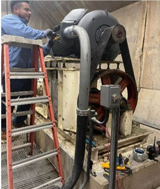
(photo above left) Dario Lopez, Electrical/Instrumentation Technician I, wiring the new motor.
