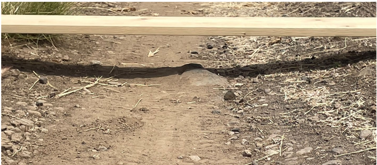
Figure 3 - Example of rutting along access road.
