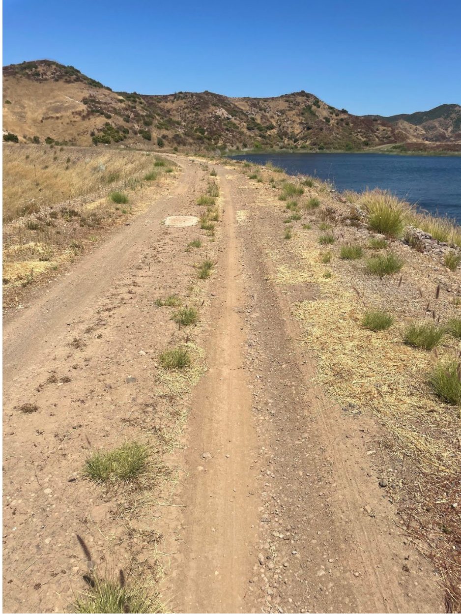
Figure 1 - Access road along crest of Westlake Dam.
