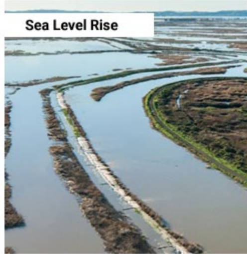
Roaring River levees overtop at Grizzly Island in Solano County located in the Sacramento-San Joaquin River Delta (Photo: Department of Water Resources)
