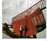
ASR-11 Air traffic control radars at LAX, 25kW peak, 2.1 kW average Safe power density level at 43 feet
