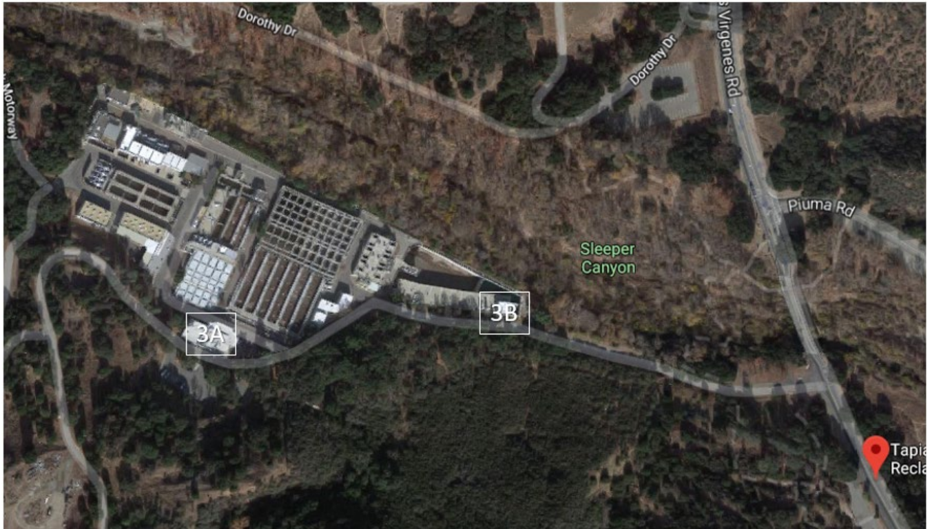
Tapia Water Reclamation Facility – 731 Malibu Canyon Road
