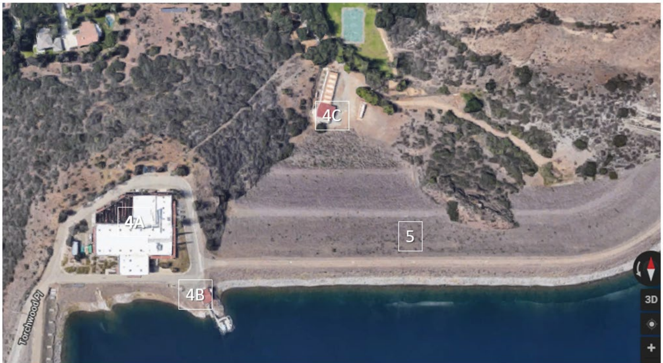
Westlake Filtration Plant and Dam - 2860 Three Springs Drive
