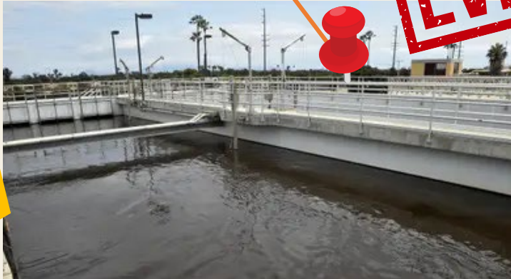
City of San Buenaventura re: Ventura Water Reclamation Facility
