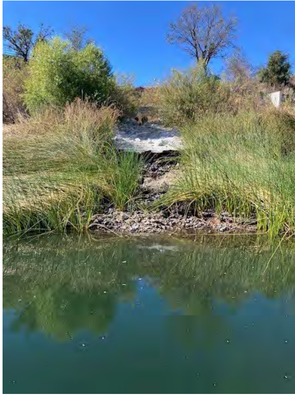
Photo 3 – Spillway Riprap
