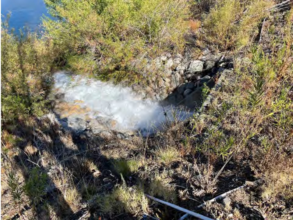
Photo 2 – Outlet Structure and Spillway
