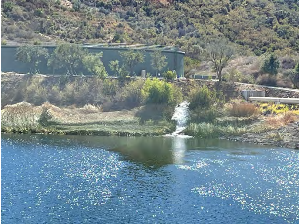
Photo 1 – Torchwood Tank, Outlet Structure, and Spillway
