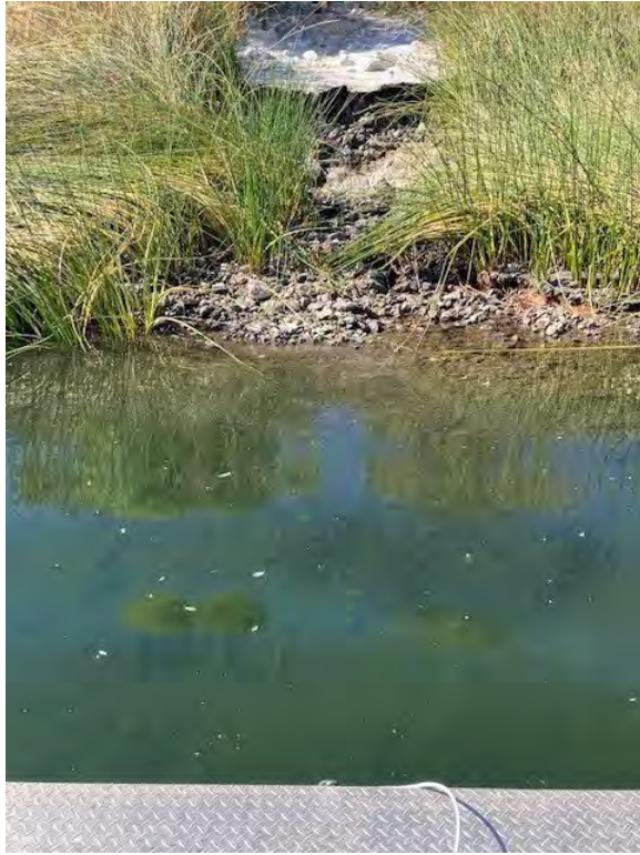
Photo 7 – Spillway Riprap limits
