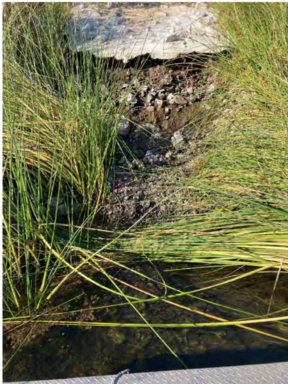
Photo 8 – Spillway Riprap limits
