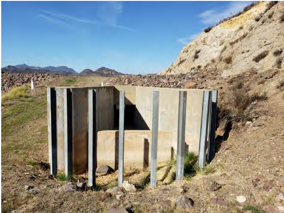
The approach to the spillway was clear.
