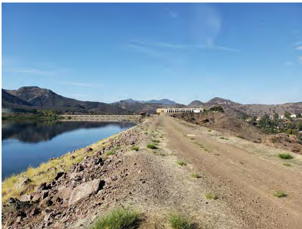
The upstream slope of the Main Dam.
