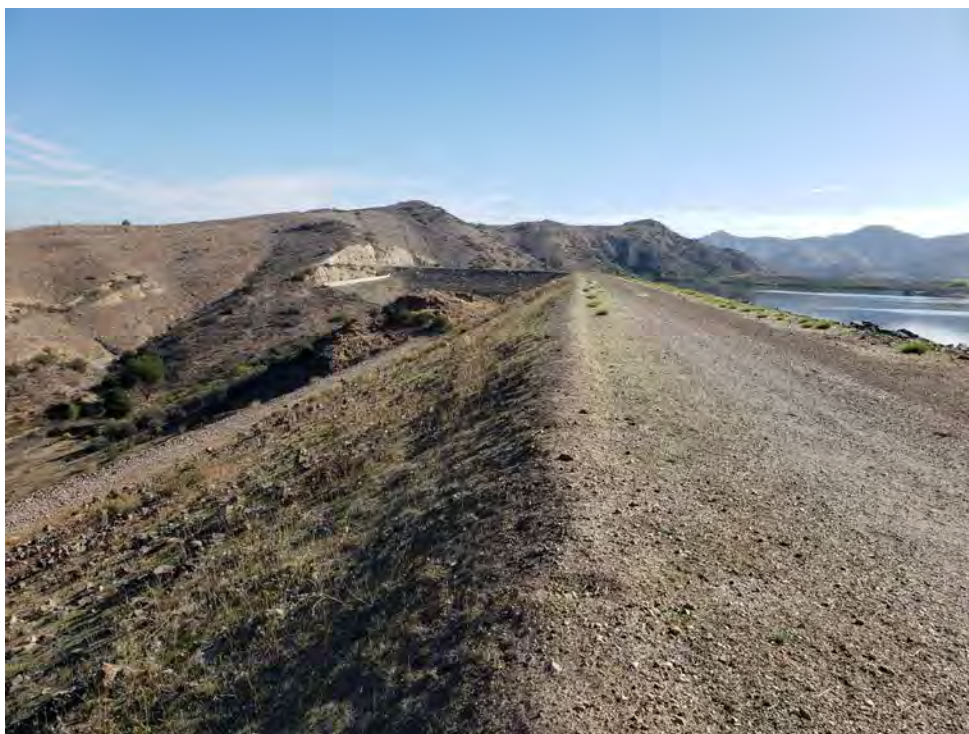
The crest and downstream slope of the Main Dam.
