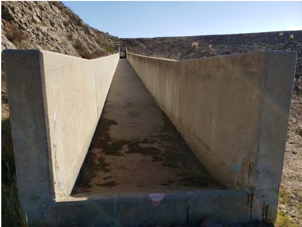
End of the spillway channel looking upstream.
