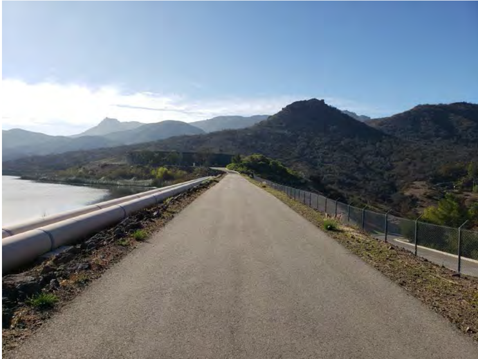
Looking down the crest of the Saddle Dam.
