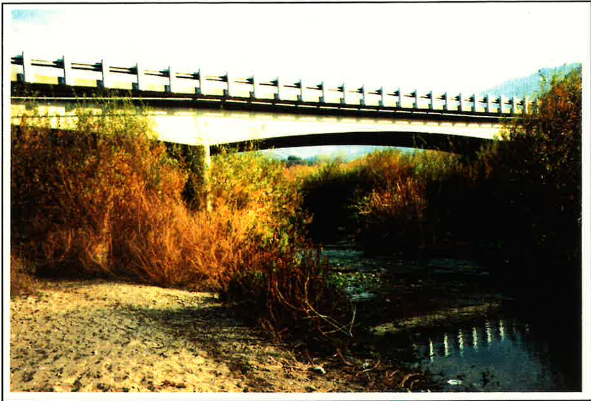
Figure 4.2 Malibu Canyon Road Bridge Looking Downstream
