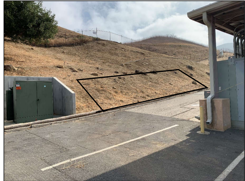
d. Battery storage system site at Recycled Water Pumping Facility
