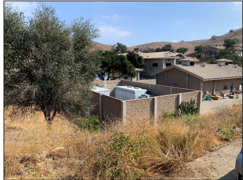
b. Electrical enclosure at the Composting Facility (new battery site)
