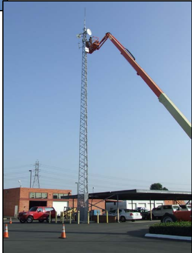
Figure 3-2 Backhaul Antenna Installation and Mast
