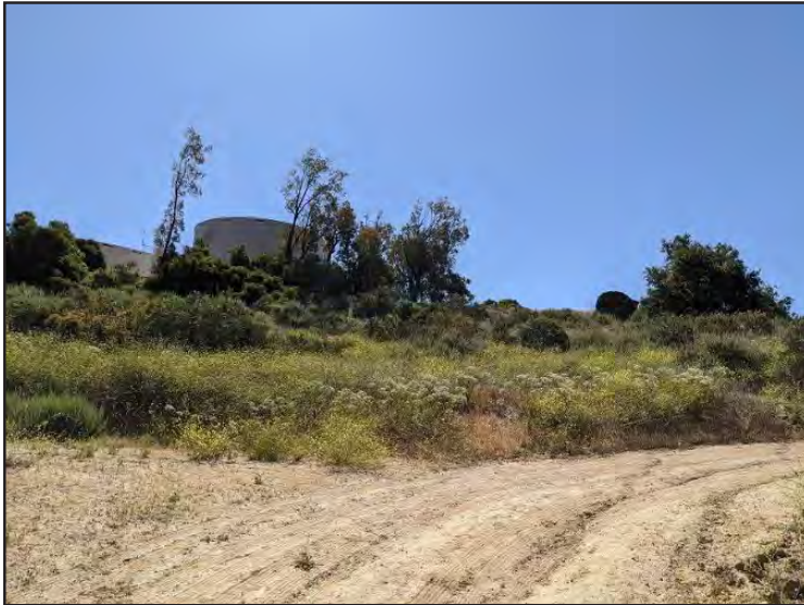
Photo 1A – Looking east toward existing water tank area along access road. The existing tower area has been lined with planted trees, primarily eucalyptus species. Photo taken May 10, 2020.
