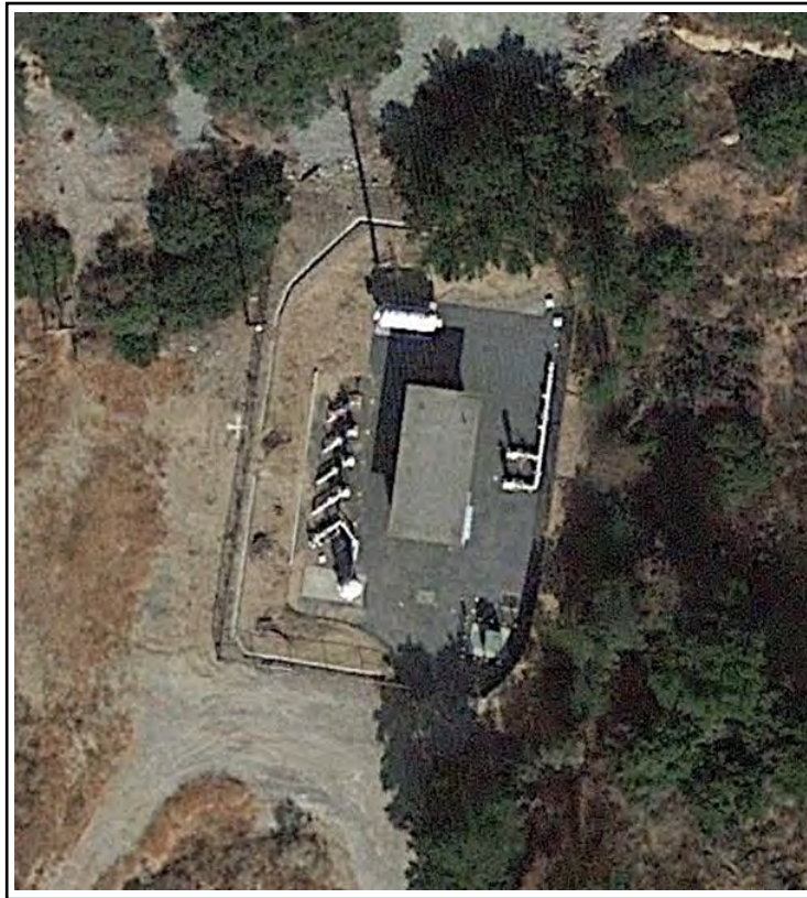
Photo A – Existing conditions image of the Twin Lakes Pump Station as currently developed. Aerial Imagery: GoogleEarth Pro, Dec. 31, 2017.
