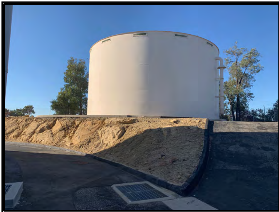
Figure 9: Project development footprint showing the Water Tank to be replaced.
