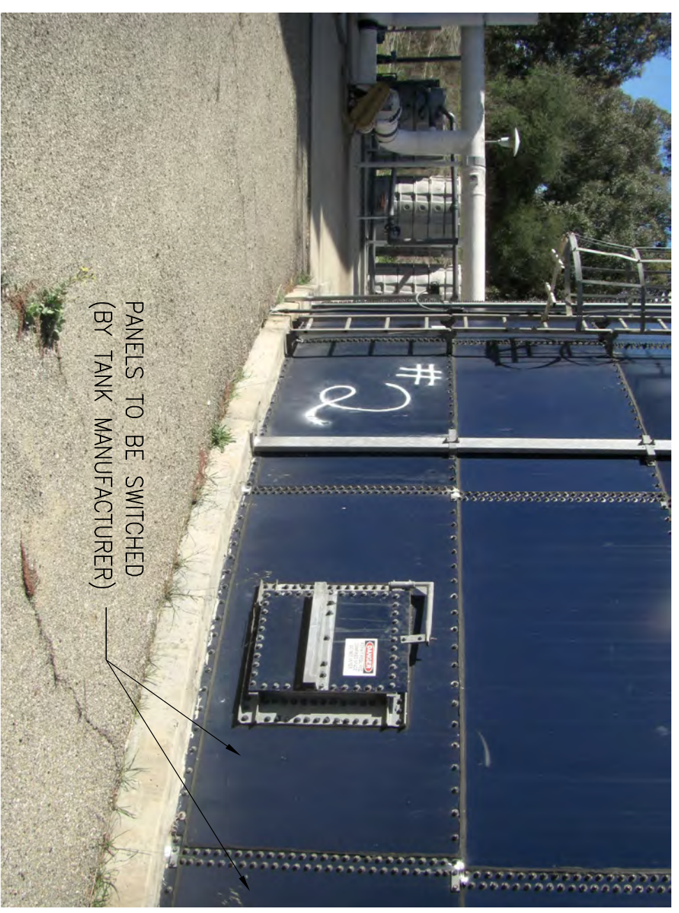
TANK NO. 2 MODIFICATIONS SCALE: NTS
