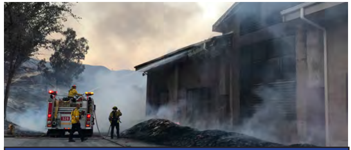
The Woolsey Fire caused significant damage at the Rancho Las Virgenes Composting Facility.
