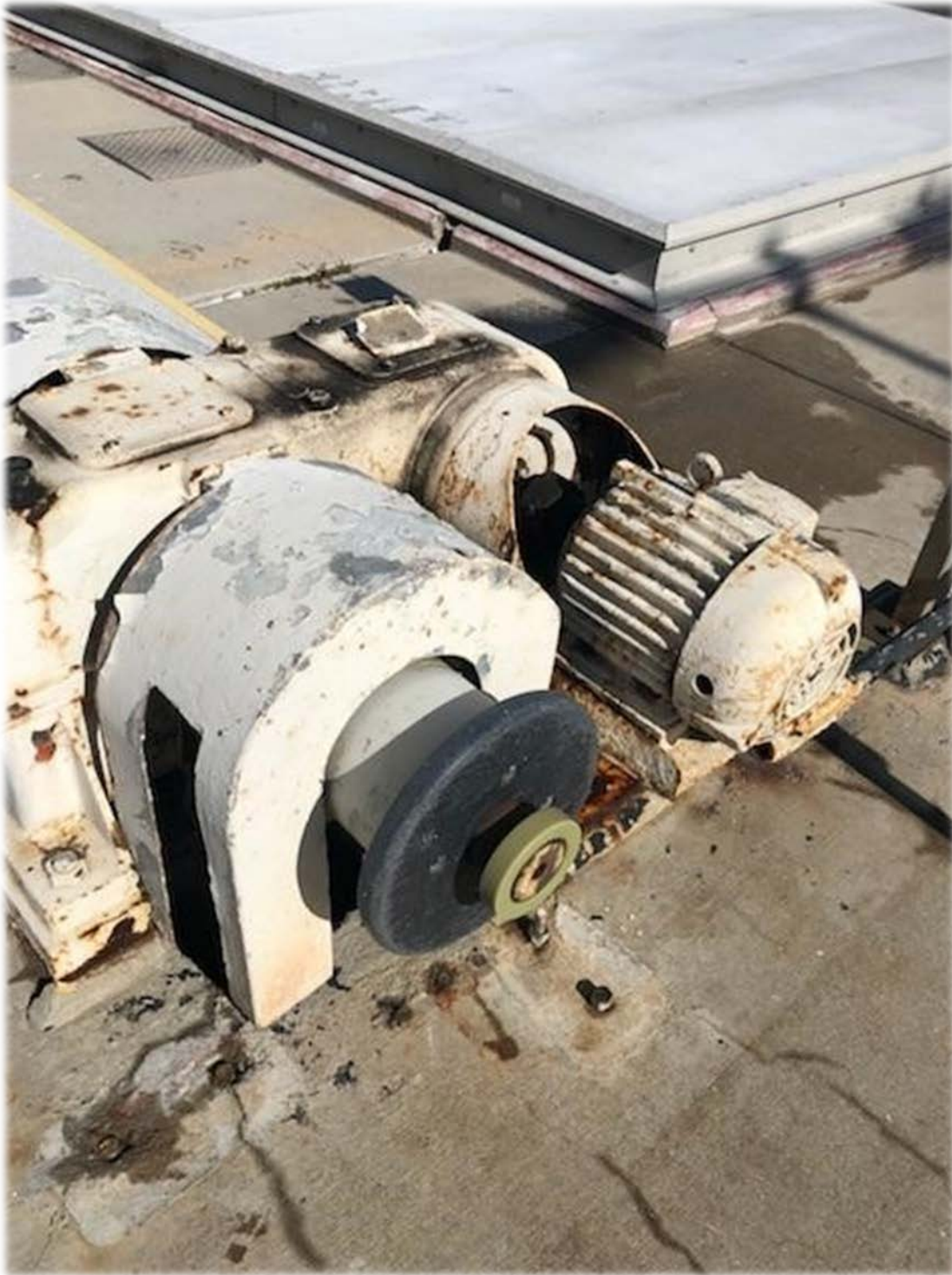
Existing Drive for Primary Scum Collection System
