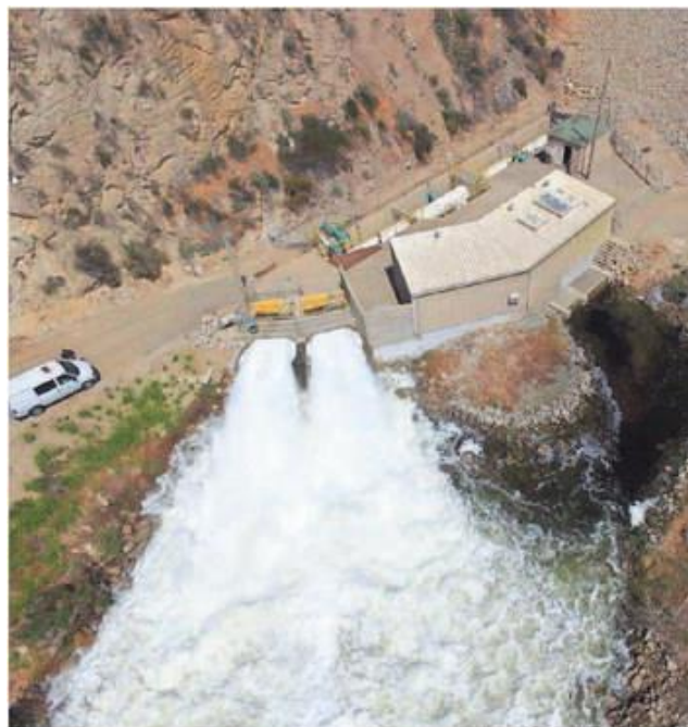
Water is released from the Santa Felicia Dam at Lake Piru in June 2017. The dam captures runoff from the rainy season and it is then released in late summer or fall to provide groundwater. UNITED WATER CONSERVATION DISTRICT PHOTO
