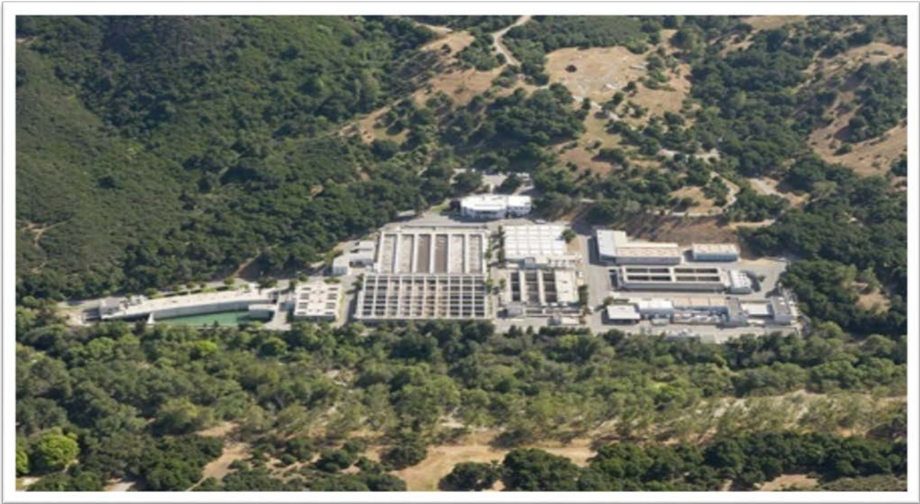
Tapia Water Reclamation Facility Operated by Las Virgenes-Triunfo Joint Powers Authority
